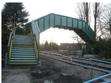
Typical 'up and over' half-through plate girder
